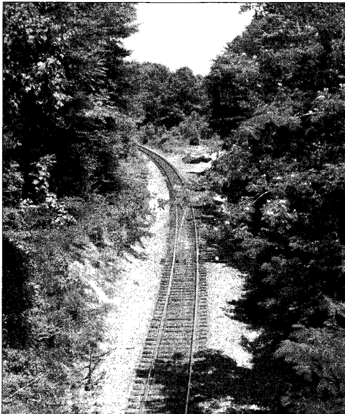
View North of Commuter Rail Line in Proposed Station Area
